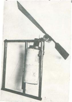
FIG. 10 No. 23 steam operated twin cylinder rotary engine built to power the 1896 aeroplane<sup>7</sup> showing steam boiler and tubular frame which also served as a container for water and kerosene for the operation of the boiler. Engine built in 1898
